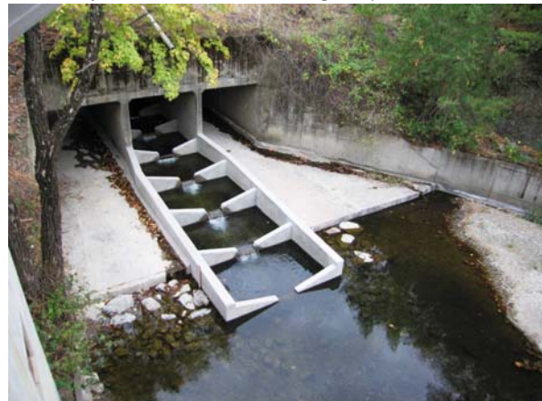
After: Box Culvert with Pool & Chute Fish Ladder
